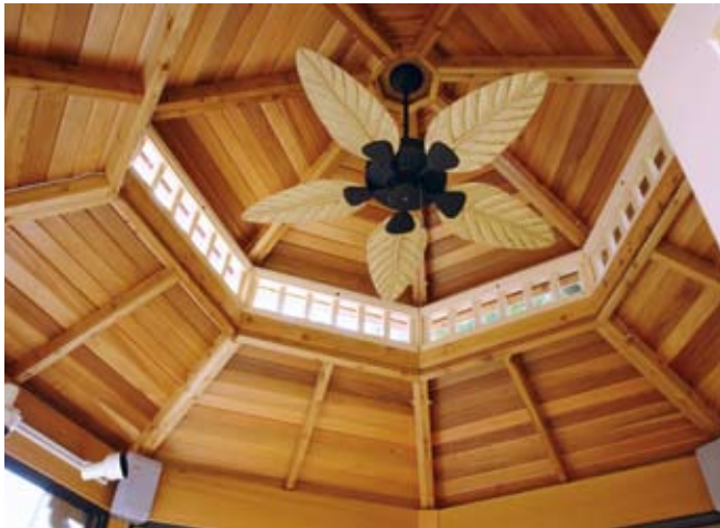
An optional 5/4 x 4 tongue and groove clear cedar ceiling graces the interior of a 12' two tier gazebo. Roof sections are bolted together with brass acorn cap nuts and brass washers.
